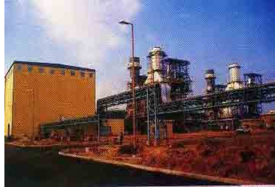
Takoradi Power Plant
