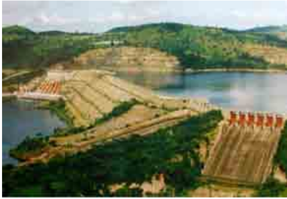
Aksoombo Power Plant
