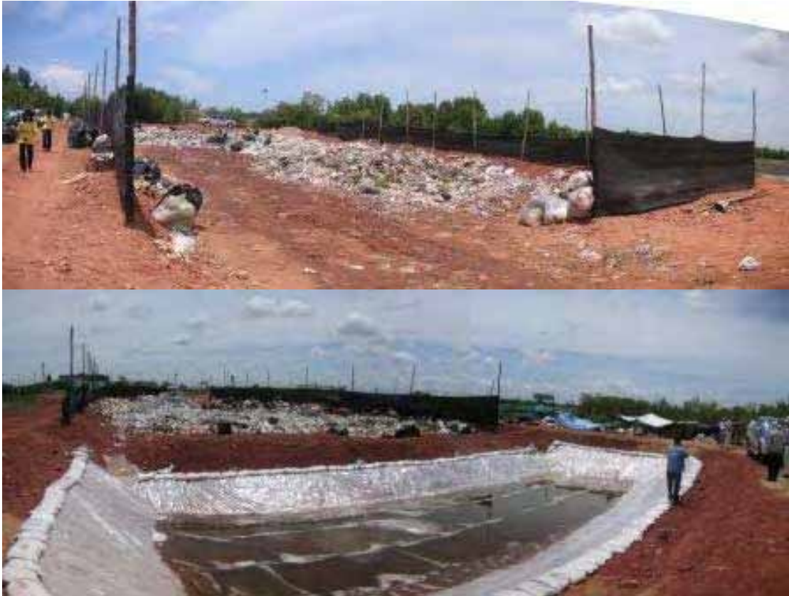
Figure 5-28: General View of Transfer Station in SKP
