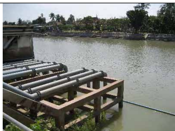
Water Purification Plant of Ayutthaya City on December 20, 2007
