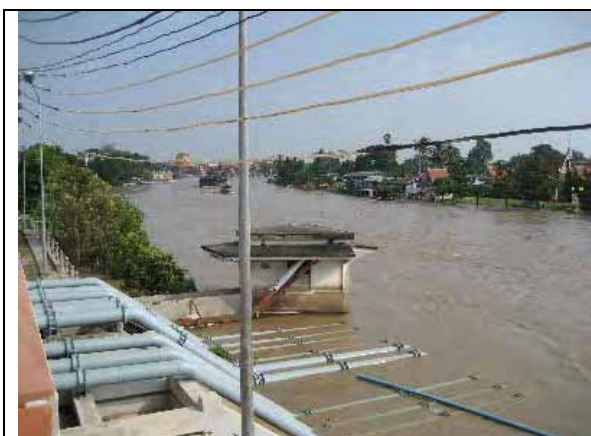
Water Purification Plant of Ayutthaya City on October 22, 2007
