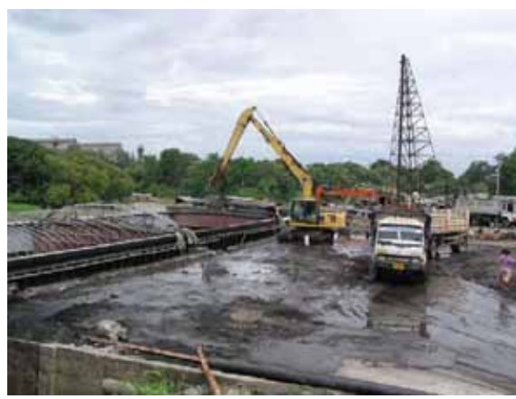
The river ports on the Chao Phraya River in AYP (with moorings for coal- and cement-carrying barges) are sources of public complaints about noise and dust.
