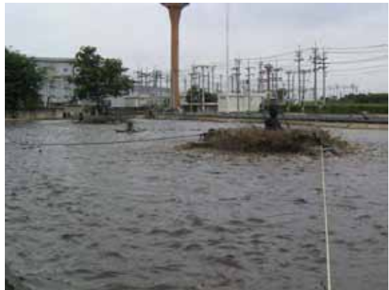
Wastewater treatment pond of Suan Autasahakham Rojana Industrial Zone, AYP. The water quality of treated wastewater met PCD standards.
