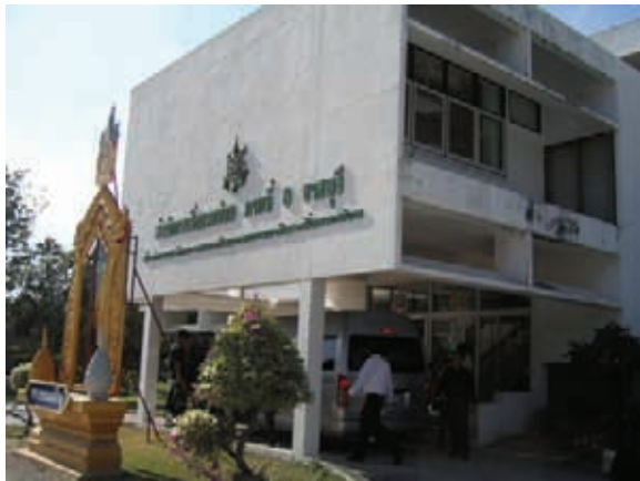
Office entrance, REO8, in Ratchaburi Province. REO8 oversees SKP.
