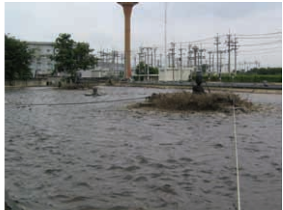
Wastewater treatment pond of Suan Autasahakham Rojana Industrial Zone, AYP. The water quality of treated wastewater met PCD standards.
