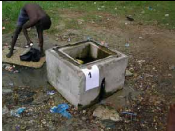
Point 1, Well (Confined Groundwater), Relatively clear water is continuously pouring.
