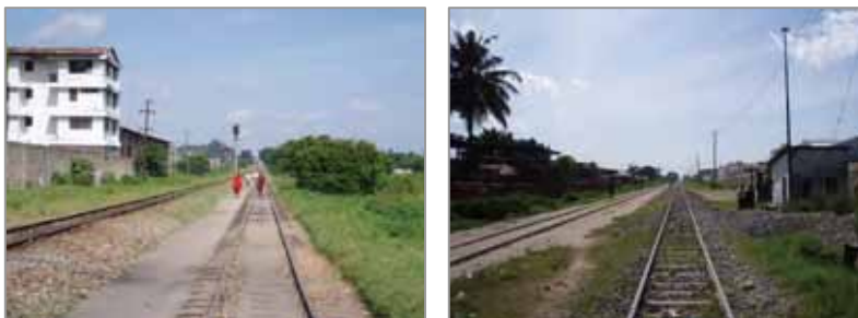
Figures 11.5.4 & 11.5.5 Showing unused rail corridor along Buguruni Section
