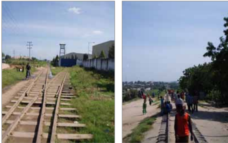
Figures 11.5.6. & 11.5.7 Showing deviation into potential BRT depot site at Ubungo and a narrow section along the Tabata section
