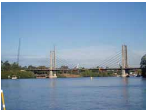
Figure 7.5.8 Brisbane Green Bridge
