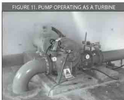
FIGURE 11. PUMP OPERATING AS A TURBINE
