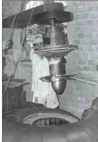
FIGURE 13. KAPLAN AND PROPELLER-TYPE TURBINE
