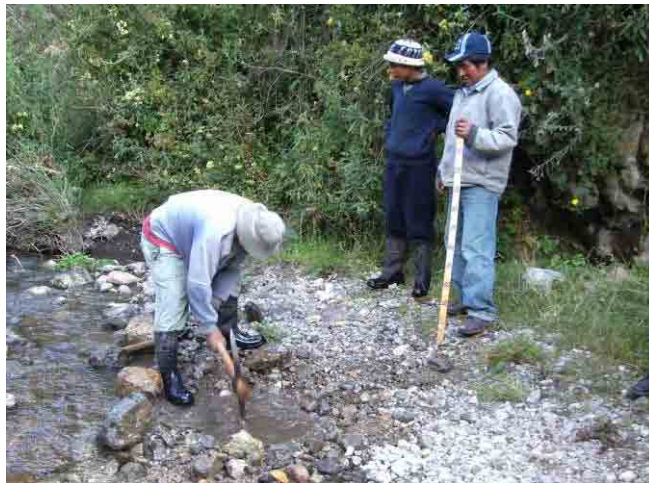
Photo III-3.5.1-7 Situation of Staff Gauge Installation
