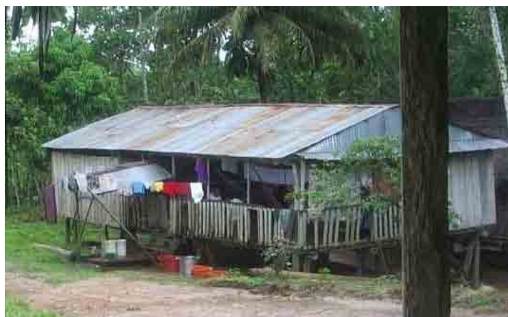
Photo III-2.5-3 Open Structure of Typical Household
