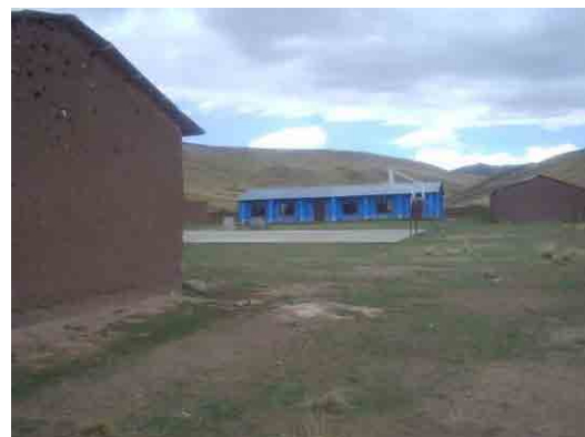
School building being used: building 1 (front), 2 (back)
