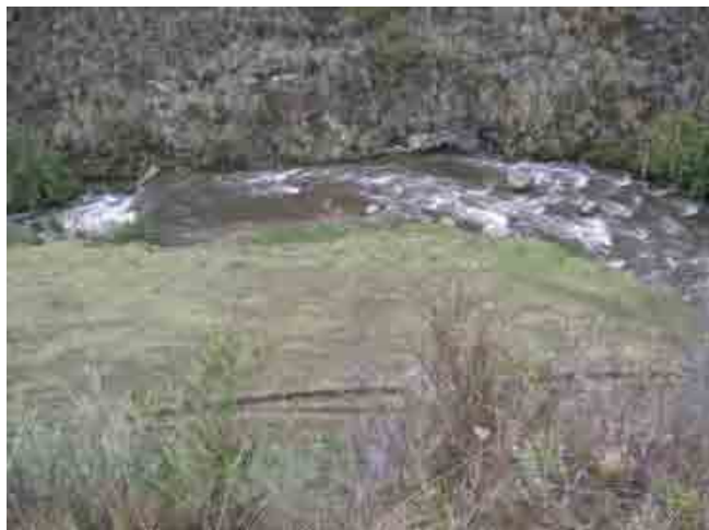
Photo III-3.5.1-19 Planning site of Powerhouse
