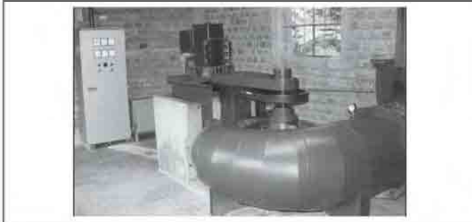
FIGURE 22. 5 KW AXIAL TURBINE WITH A HORIZONTAL HUB AND A 4:1 BELT AND PULLEY TRANSMISSION SYSTEM
