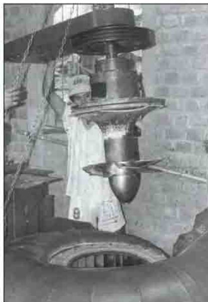
FIGURE 13. KAPLAN AND PROPELLER-TYPE TURBINE
