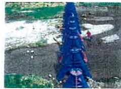
Anticorrosive coating of Slit-dam
