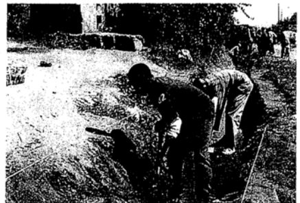
Volunteers digging drainage in Chipata
