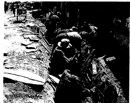
Volunteers laying flat stones for drainage
