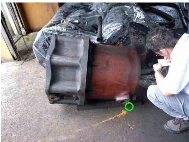
Cooling water jacket (green circle indicates the cracked area)
