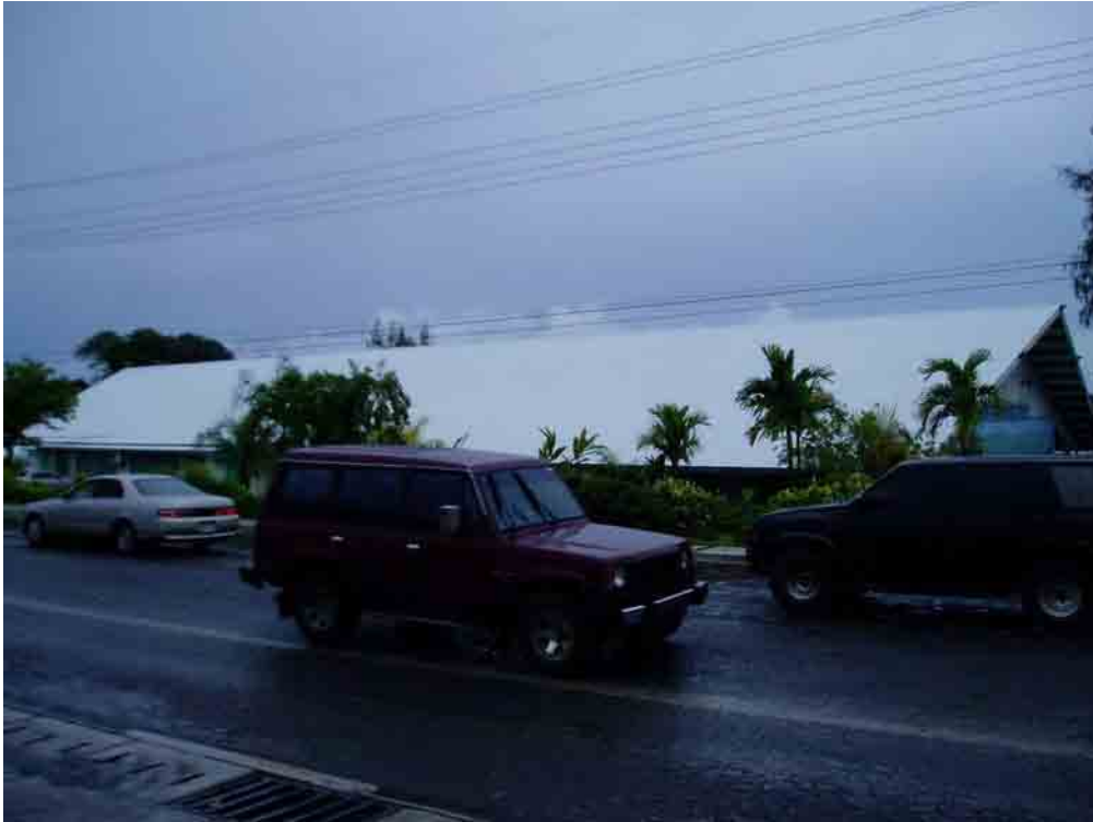
Fig. 4.3.2-1 Gymnasium of Palau Community College
