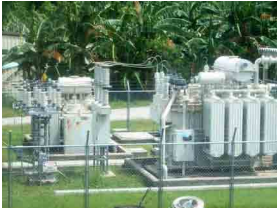
Fig. 2.4.2-1 Malakal Power Plant
