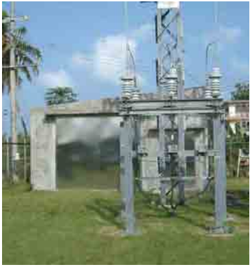
Fig. 2.4.2-9 Airai Substation (building)
