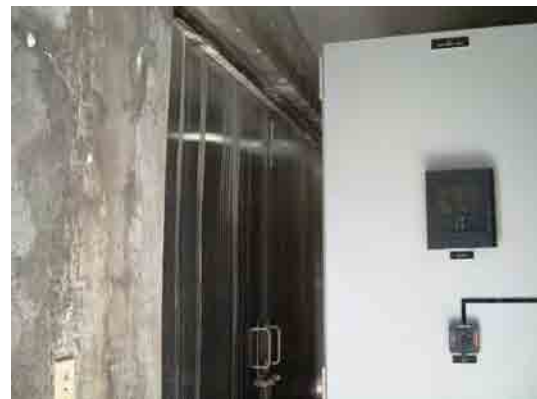
Fig. 2.4.2-19 Equipment Delivery Door
