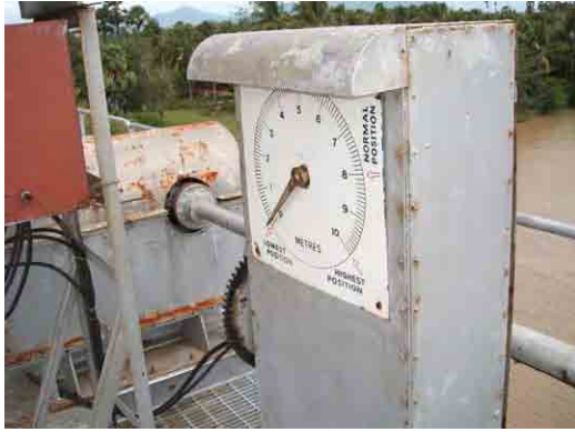
Position Indicator does not function.
