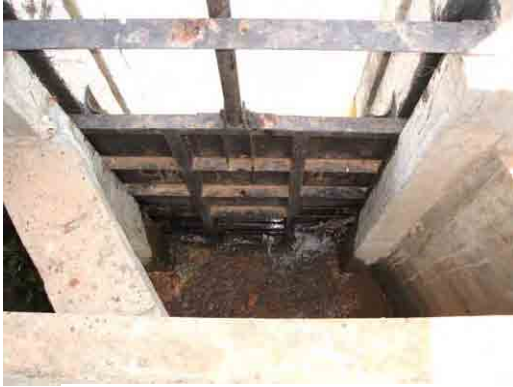
No Provision of Metal Seal Seat
