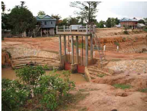
Unnecessarily Long Spindle
