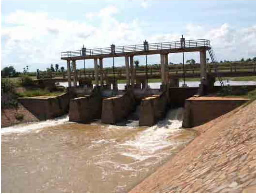
View from Downstream
