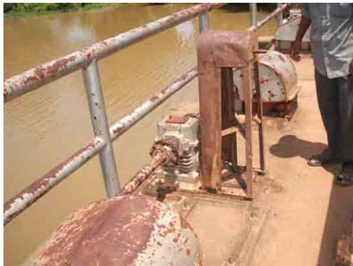
Removal of Electric Motor and Control Panel
