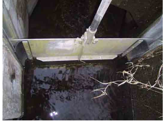
Example of Stainless Steel Seal Seat
