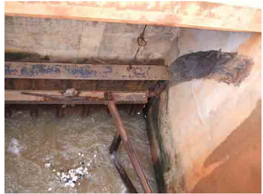
Temporary Measure for Wire Rope
