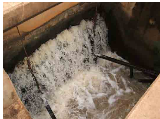
Temporarily Hoisting Wire
