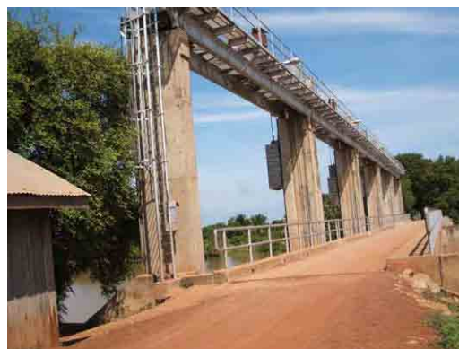
Downstream of Pier
