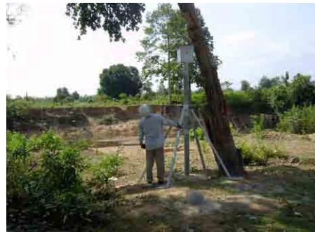
Sangkea Tasal Water Level Gauging Station
