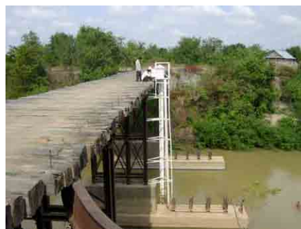
Peam Khley Water Level Gauging Station
