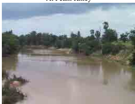
Thnuos Luong Station Site Staff gauge on the pier of Kampong Speu Bridge
