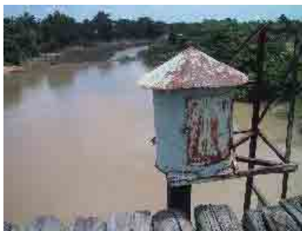
Water level gauging station with data logger At Peam Khley
