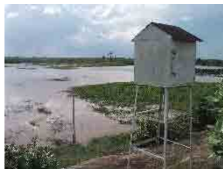
Water level gauging station at Tuk Thla Regulating Weir
