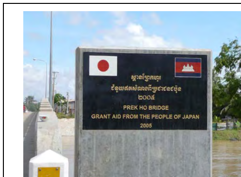
The bridge over the Prek Ho Channel at the bifurcation site
