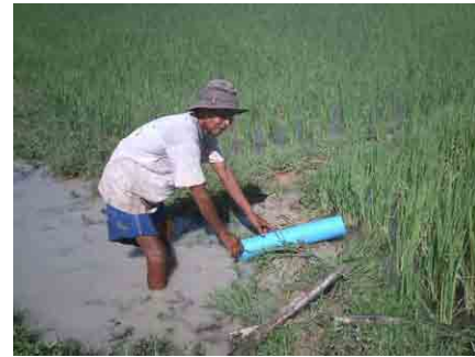
Installation of PVC pipe
