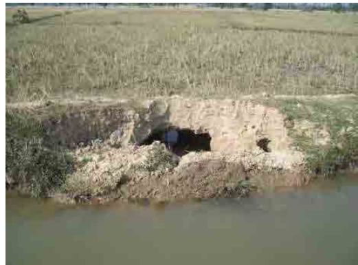
Farmers were taking water directly from the RT-2 tertiary canal by making holes
