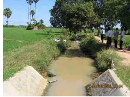
No water flow in the RT-2 tertiary canal in beginning of September 2006
