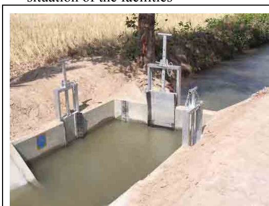
Division box with check at Bos Ta Ney village (upstream view)
