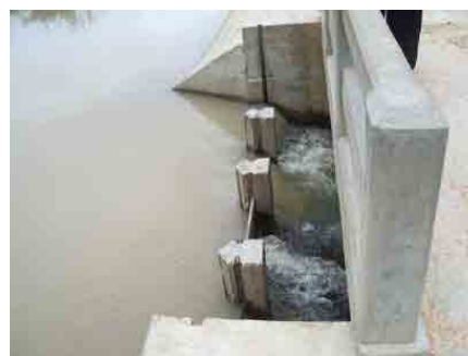
Water was flowing out from the spillway
