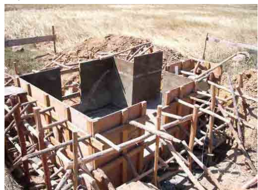
Division box under construction at Pongro village
