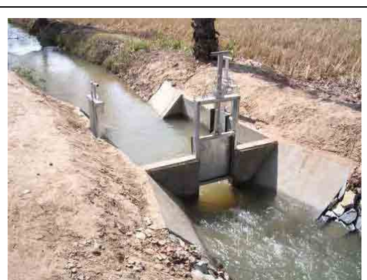
Division box with check at Bos Ta Ney village (downstream view)
