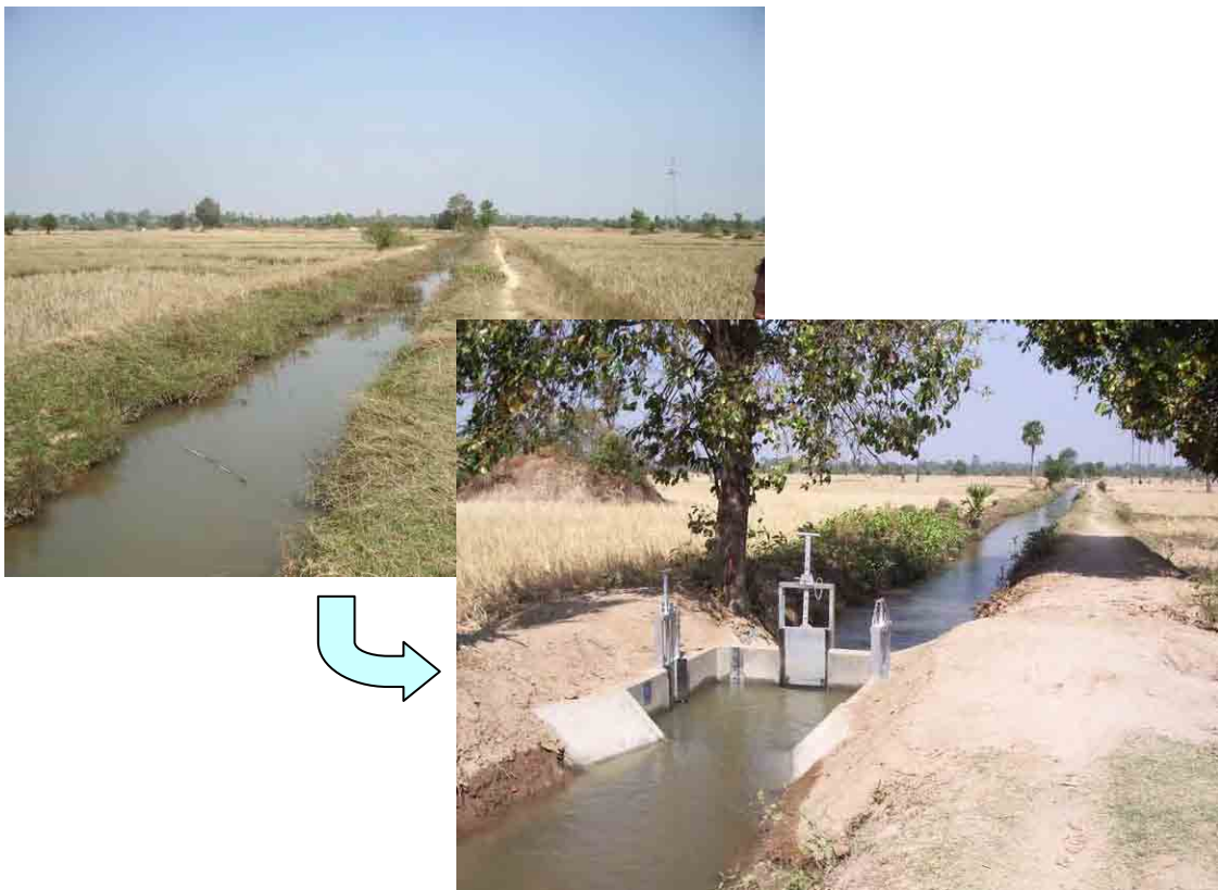
Improved Target Tertiary Canal (RT-2 Canal) (Participatory Irrigation Management and Development Activities in Zone-1)
