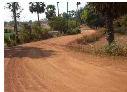
Earthen road near the Project Site
