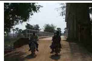
Passage on maintenance bridge of Roleang Chrey Regulator
