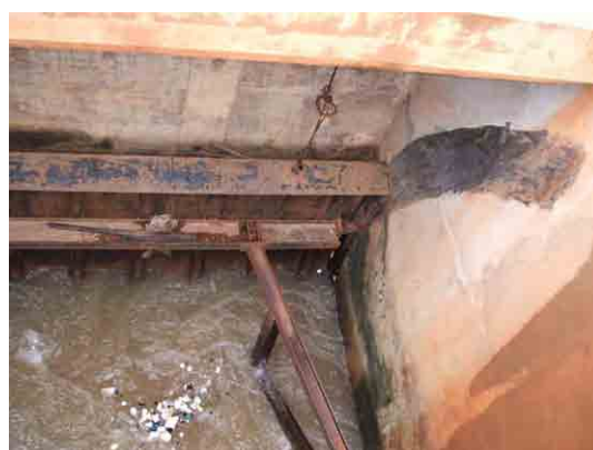
Temporary Measure for Wire
