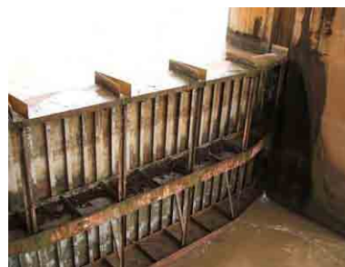
Downstream View of Gate Roleang Chrey Regulator
