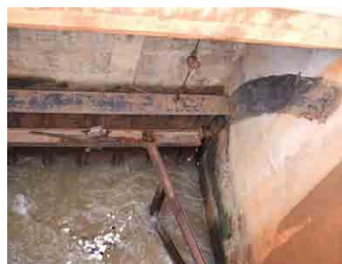
Temporary Measure for Wire Rope
