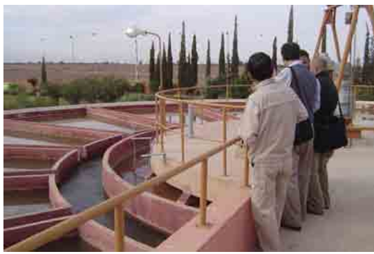
Potable Water Treatment Facility near Marrakech
