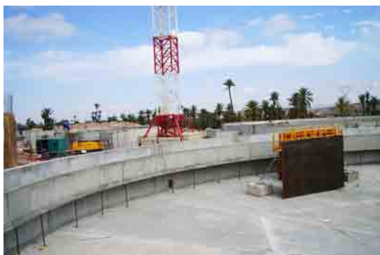
Sewage Treatment Plant under Construction
