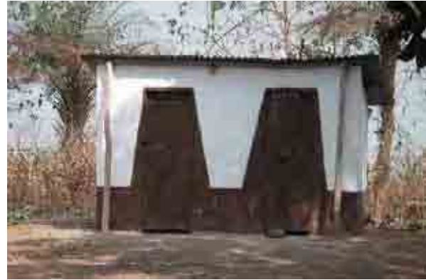
Figure 4.11: School Toilet Constructed (B11)
