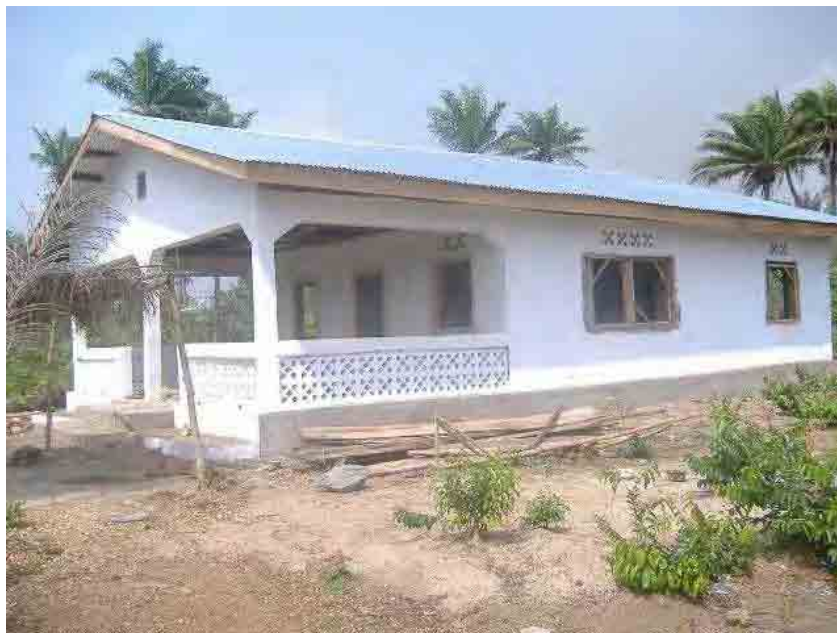
Figure 4.3: Constructing a Health Post (M10)
