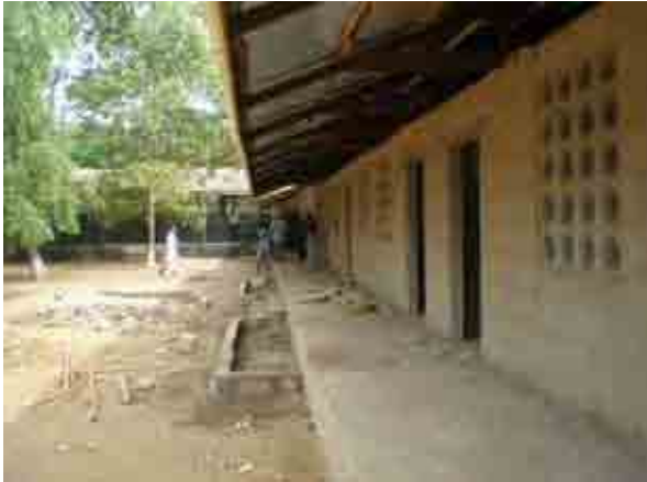
Figure 4.2: Cement Mortar in Concrete Block (M01)
