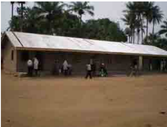
Figure 4.1: Cement Mortar in Concrete Block (M02)
