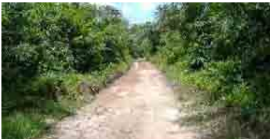
Figure 4.4: Rehabilitated Road (T07)
