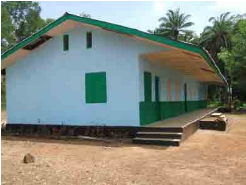
Construction of 3 Classrooms
