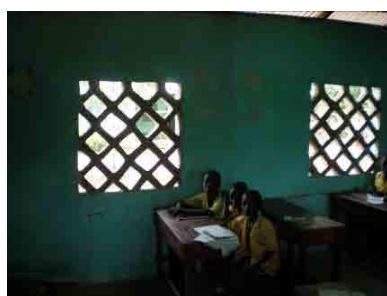
Ventilation Block by Wooden Mold in Step 2
