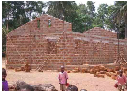
Figure 3.35: Cement Mortar in Block Joint (M06)
