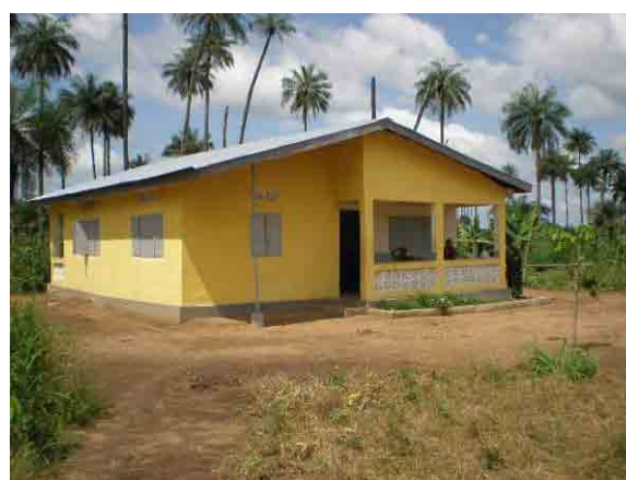
Figure 3.31: Construction of Staff Quarters Completed (B10)
