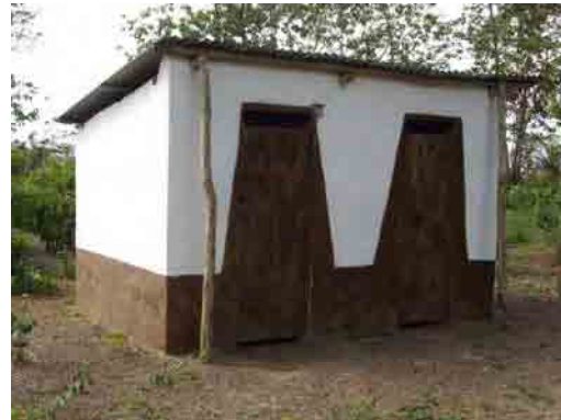
School Toilet Construction
