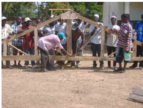
Figure 2.40: Truss Fabrication
