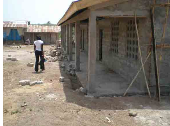
Figure 3.42: Change to Reinforcement Concrete Structure (T01)
