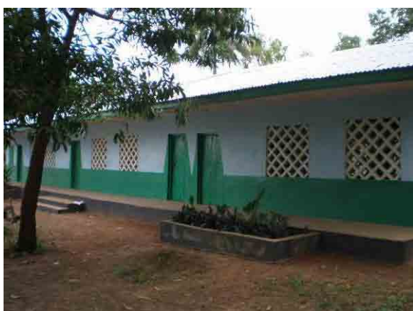
Figure 3.30: Construction of 3 Classrooms and Office with Store Completed (M06)
