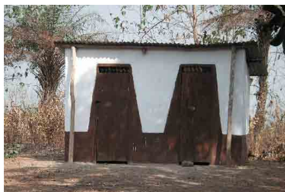
Figure 3.27: School Toilet Constructed (B11)
