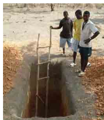
Figure 3.4: A Pit for a School Toilet (T08)
