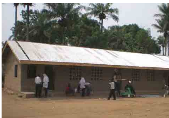
Figure 3.36: Cement Mortar in Concrete Block (M02)
