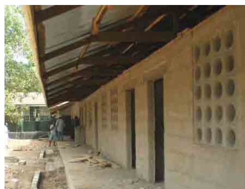
Figure 3.37: Cement Mortar in Concrete Block (M01)
