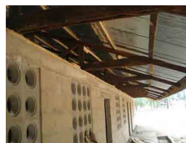
Step 3 Ventilation Block by Steel Mold for Classroom
