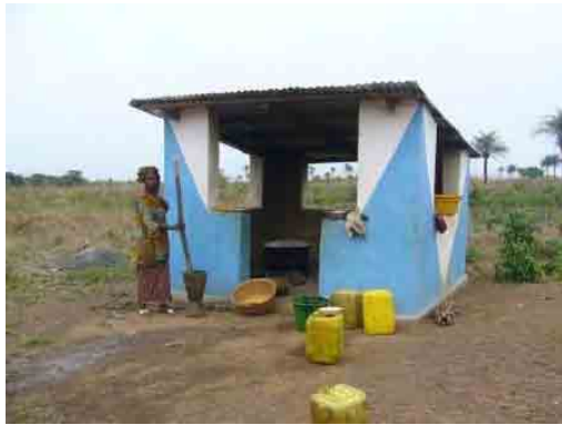
School Kitchen Construction
