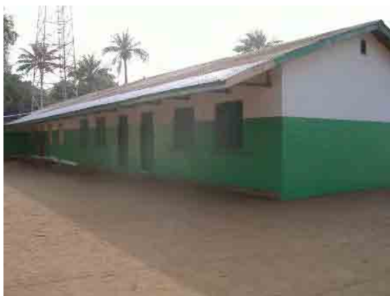
Figure 3.9: School Building Rehabilitated without Technical Support (M02)
