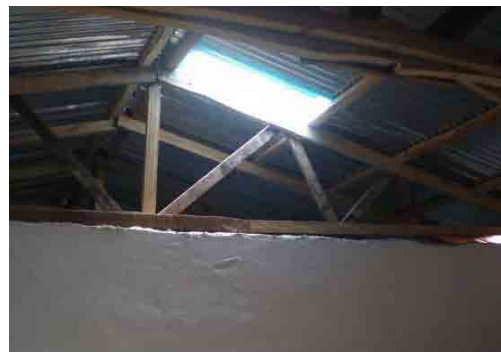
Figure 3.38: Transparent Sheet in Roof for Light (T05)
