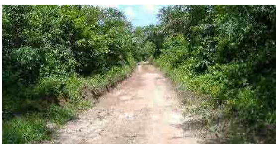
Figure 3.23: Rehabilitated Road (T07)
