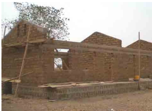
Figure 3.34: Mud Mortar in Block Joint (B03)
