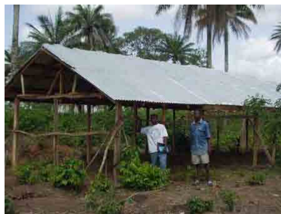
Figure 3.10: Temporary Shed (M12)
