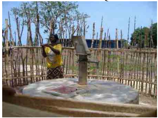
Rehabilitation of Well
