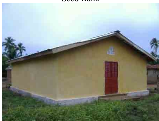
Construction of Community Seed Store
