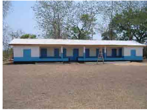
Rehabilitation of Classrooms
