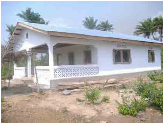
Figure 3.32: Health Post Under Construction (M10)
