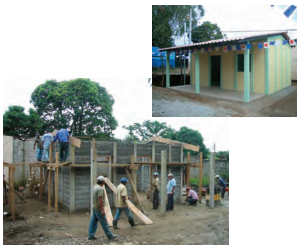
Construction technology trainees constructing an earthquake-resistant popular model house
