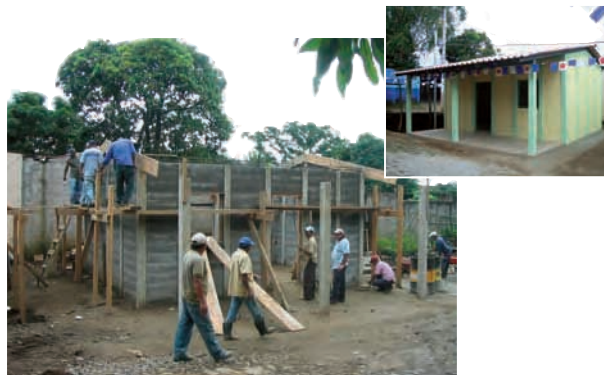
Construction technology trainees constructing an earthquake-resistant popular model house
