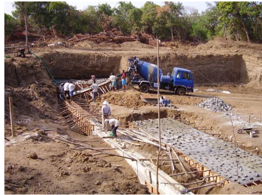
Construction of Pali Aru diversion weir by a contractor
