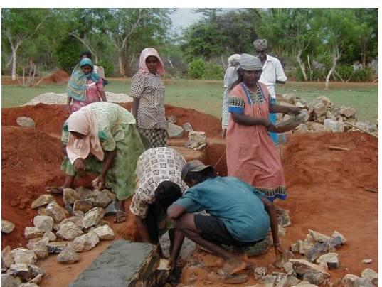
Construction of foundation for Multi Purpose Hall by CMR (Ganeshapuram)
