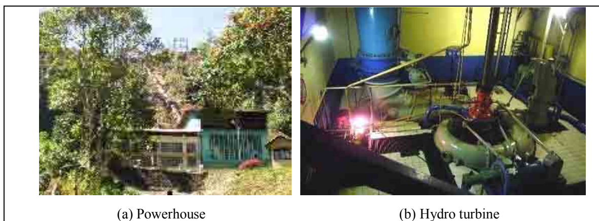
Figure 8.5.5 Current condition of Tonsealama Hydropower Station
