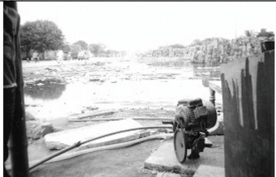
Suction pump draws water from pipeline passing through a Nala.
