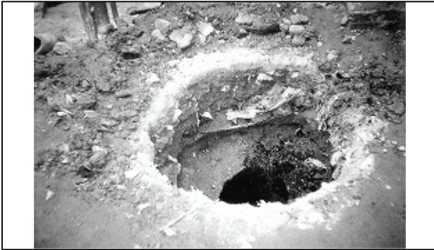
Broken gutter may cause accident.
