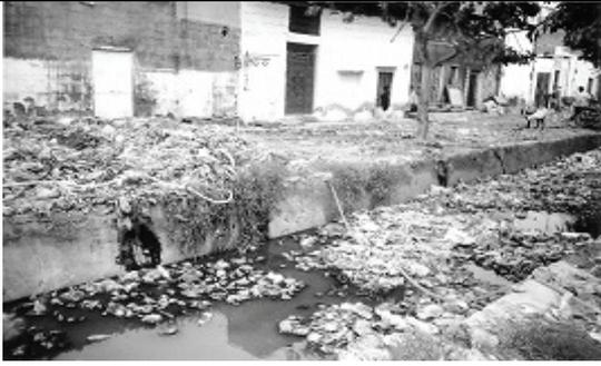
Garbage in Nala causes blockage in sewer flow.
