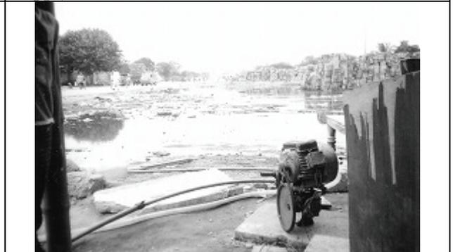
Suction pump draws water from pipeline passing through a Nala.
