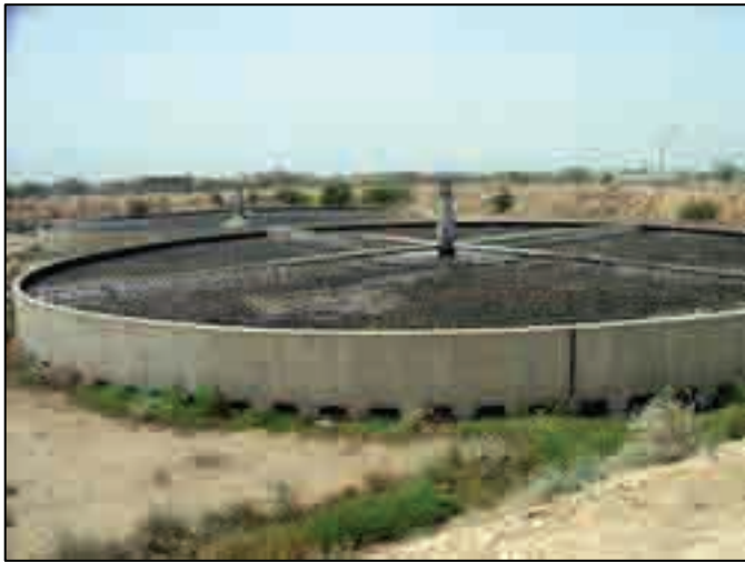
Photo 33.2.19 Trickling Filter (TP-1, in May 2006)
