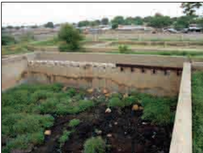
Photo 33.2.27 Final Settling Tank (North Karachi TP, abandoned)
