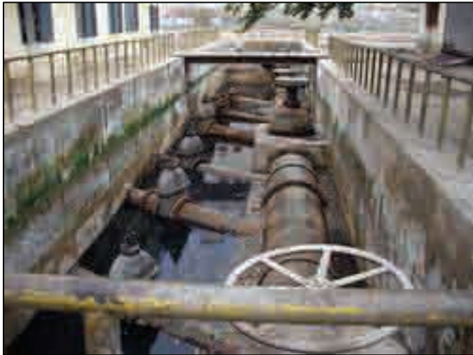
Photo 33.2.15 Discharging Pipe of Chakiwara Pumping Station
