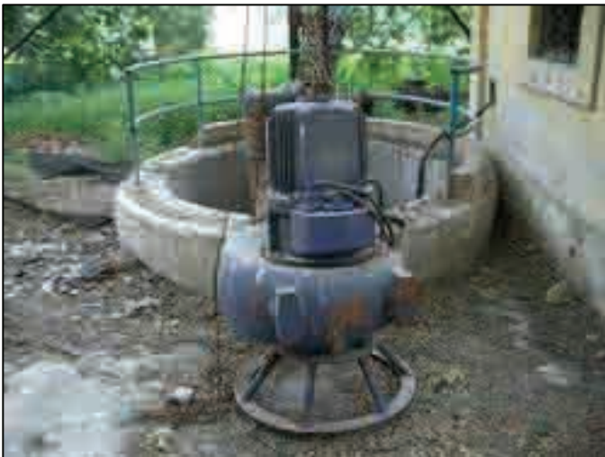
Photo 33.2.11 Submersible Pump of Jamila Pumping Station
