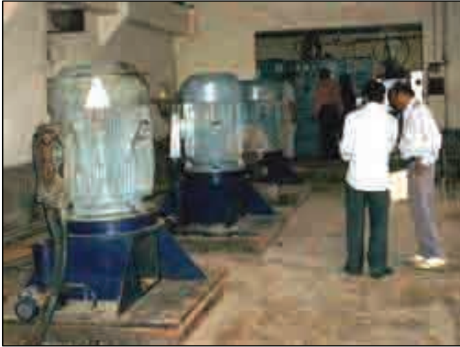
Photo 33.2.14 Vertical Type Pumps of Chakiwara Pumping Station
