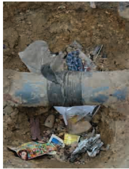
Photo 33.1.4 4" PVC Plugging with Rubber Tube
