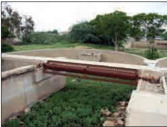
Photo 33.2.26 Oxidation Ditch (North Karachi TP, abandoned)
