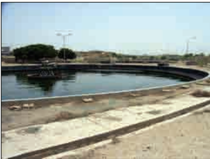
Photo 33.2.20 Final Settling Tank (TP-1, in May 2006)
