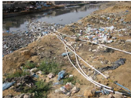
Photo 33.1.6 Piping for Illegal Connections across a Channel
