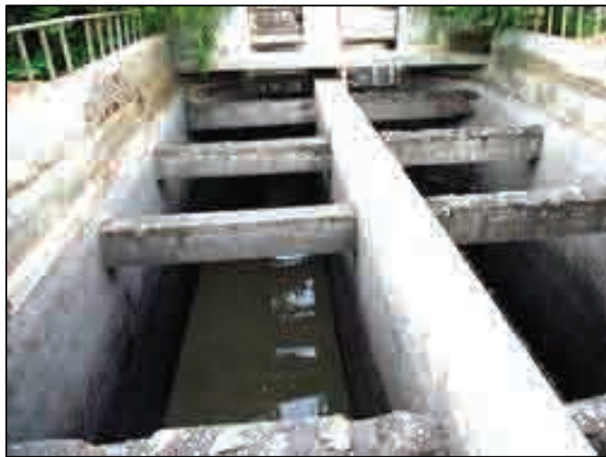
Photo 33.2.13 Grit Chamber of Chakiwara Pumping Station
