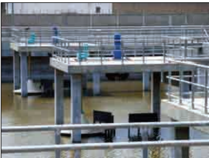
Photo 33.2.29 Both Surface and Submersible Aerator of Aeration Tank (TP of PTA)
