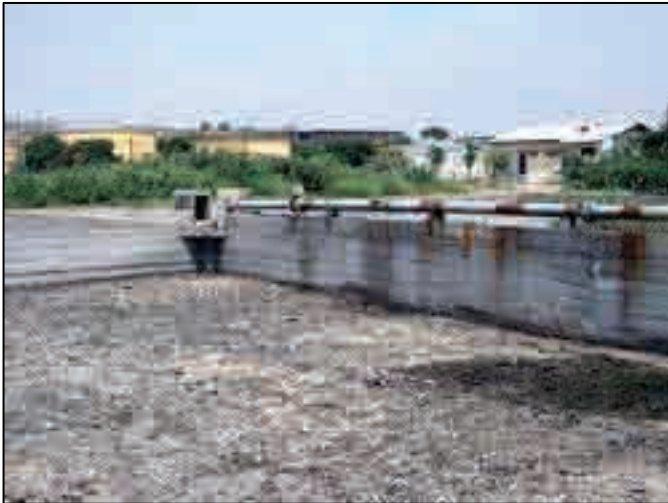
Photo 33.2.22 Sludge Distribution Pipe and Box (TP-1, September 2006)
