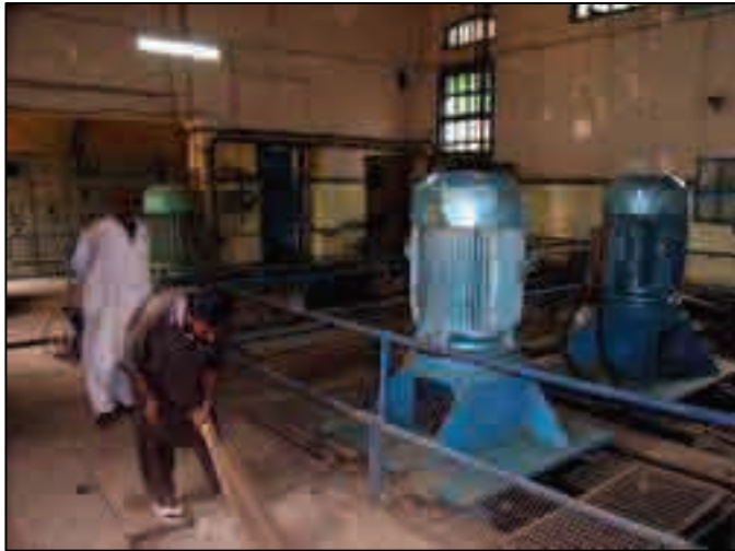
Photo 33.2.10 Vertical Pumps of Jamila Pumping Station
