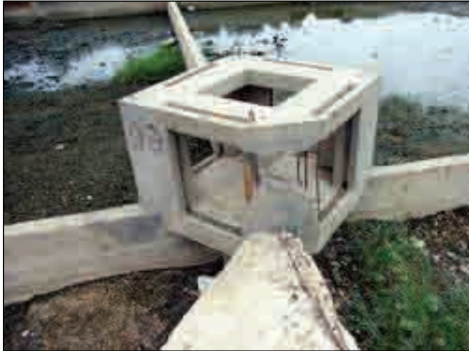
Photo 33.2.21 Sludge Distribution Box (TP-2, August 2006)
