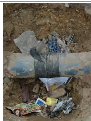
Photo S32.1.2 4" PVC Plugging with Rubber Tube
