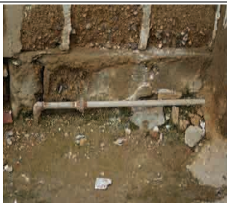
Photo S32.1.1 3/4" GIP Service Connection
