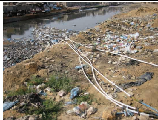
Photo S32.1.4 Piping for Illegal Connections across a Channel
