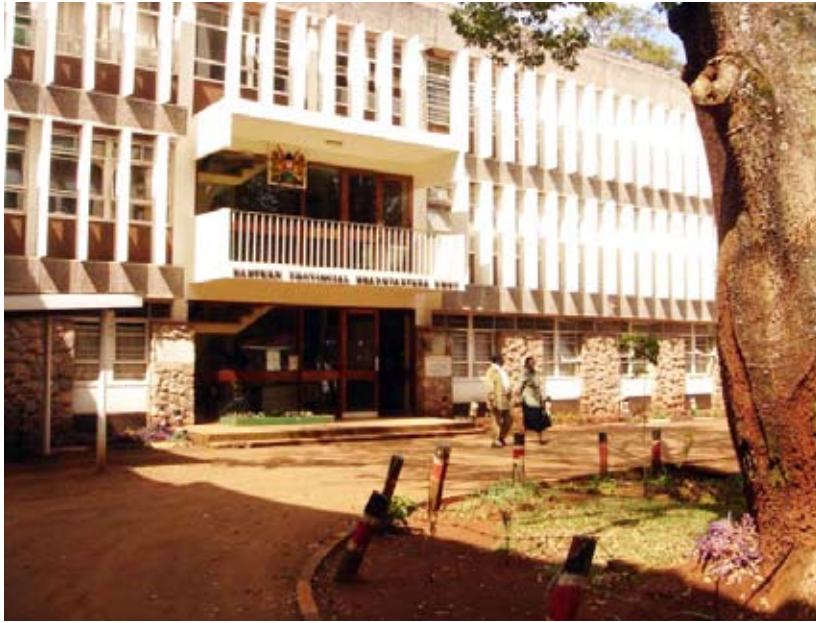
Provincial headquarters of eastern province in Embu town – its architecture a reflection of its past substantive status – significantly imposing compared to Local Authority (LA) or CDF offices.
