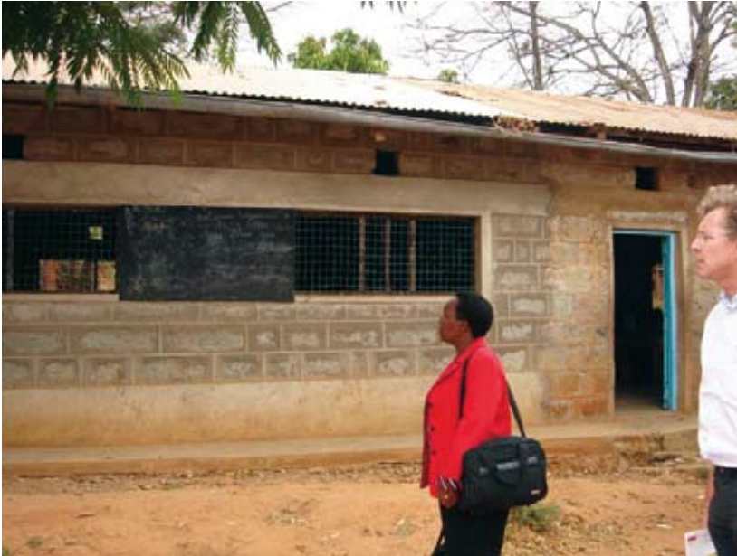
New classrooms constructed with funding from Constituency Development Fund (CDF).
