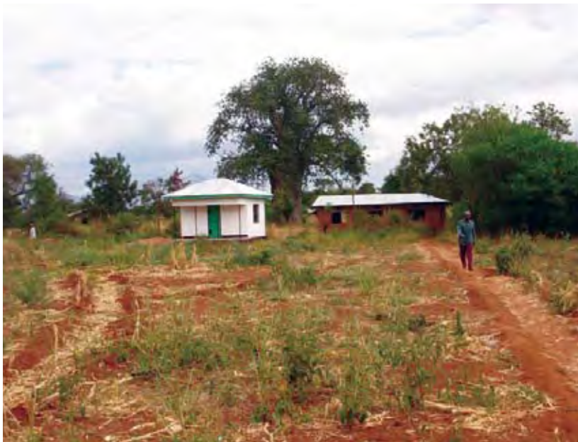
The health facility constructed in Tanzania, Moshi District – still awaiting staff and funds for recurrent costs. The missing linkages between community/ political planning (whether through Local Government (LG) structures or CDF) and technical health district planning are found in all 3 countries. While probably most significant in Kenya it is still serious in Uganda and Tanzania.
