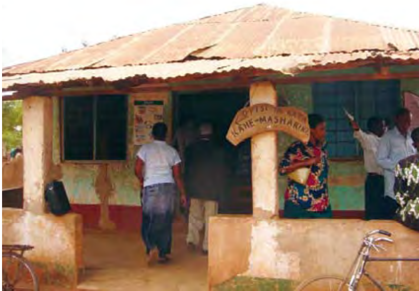
Example of the office of a Ward Development Committee in Tanzania (Moshi District).
