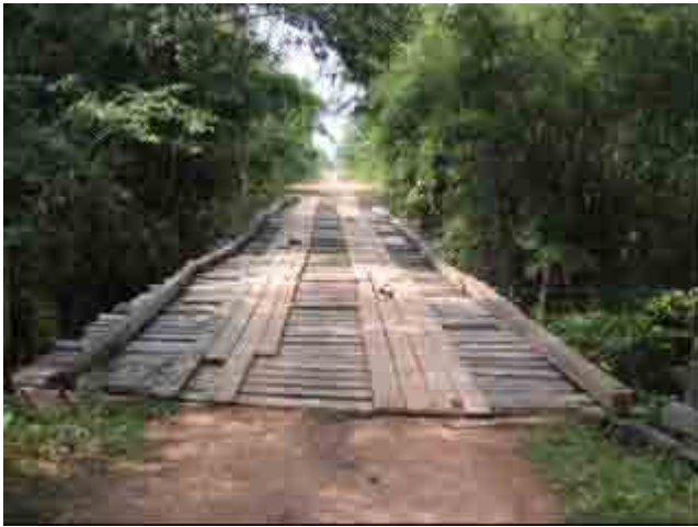
No.20+000 Doukdam Bridge
