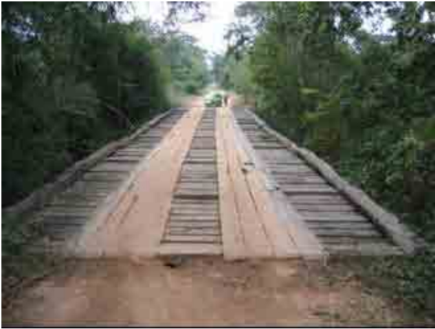
No.21+900 Ley Bridge
