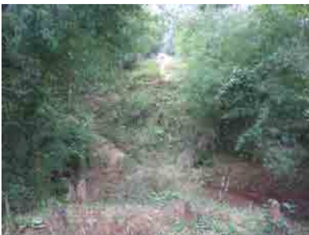
No.28+100 Pong Bridge
