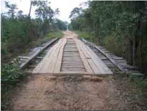
No.24+900 Phai Bridge
