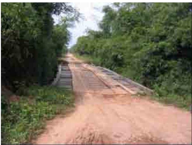
No.14+100 Dua Noy Bridge
