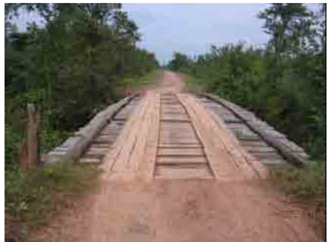
No.18+100 Bong1 Bridge
