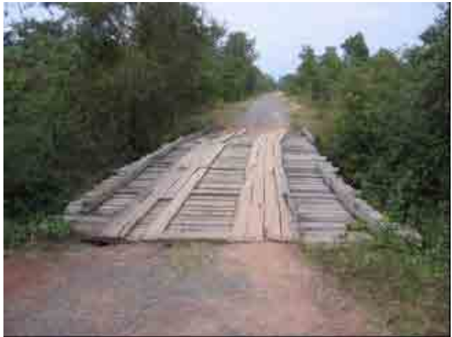
No. 12+300 Xay2 Bridge
