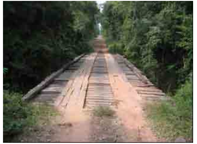
No. 20+600 Kapke Bridge
