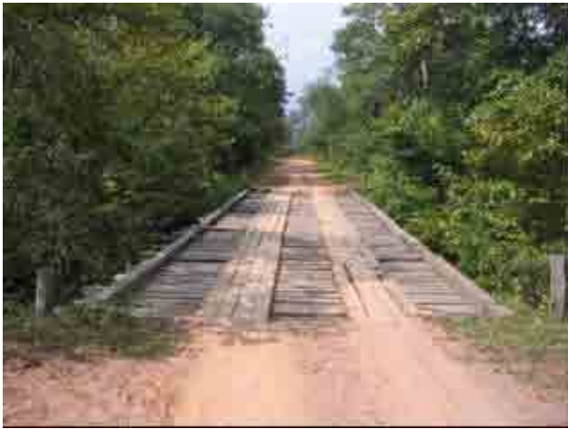
No.22+600 Kok Bridge
