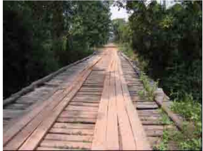
No. 23+700 Keukkek Bridge
