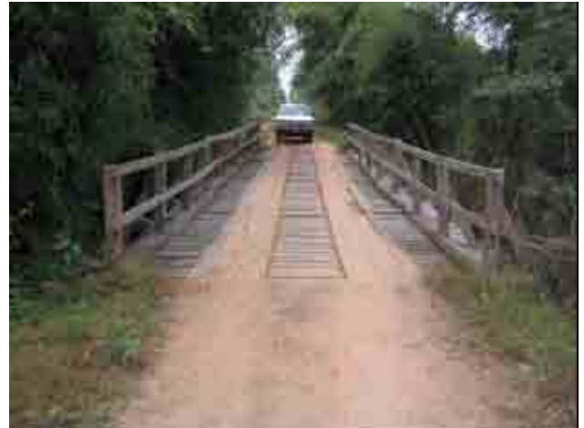
No.25+100 Sim Bridge
