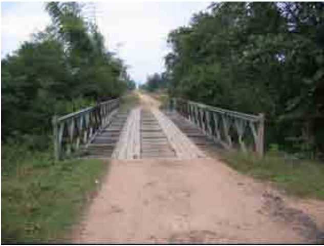
No.5+000 Xay1 Bridge (1)
