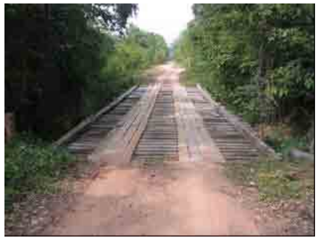
No.22+500 Mai Bridge
