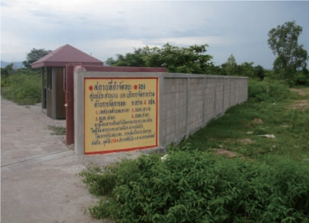
Waste treatment site supported by project
