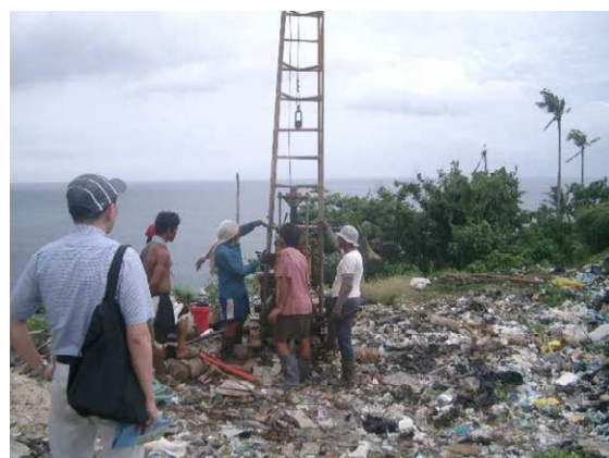
Boring for Grasping of Waste Layer Profile
