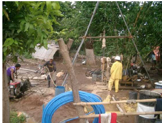
Boring of Groundwater Monitoring (No.1)
