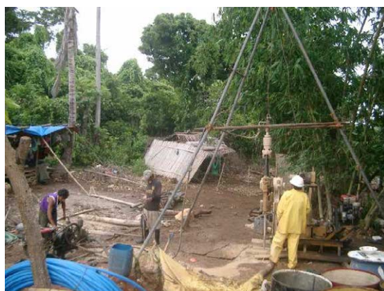
Boring for Groundwater Monitoring (No.2)
