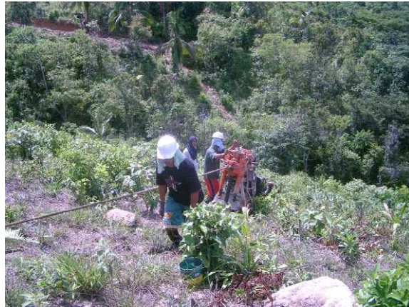
Excavation of Groundwater Monitoring Well
