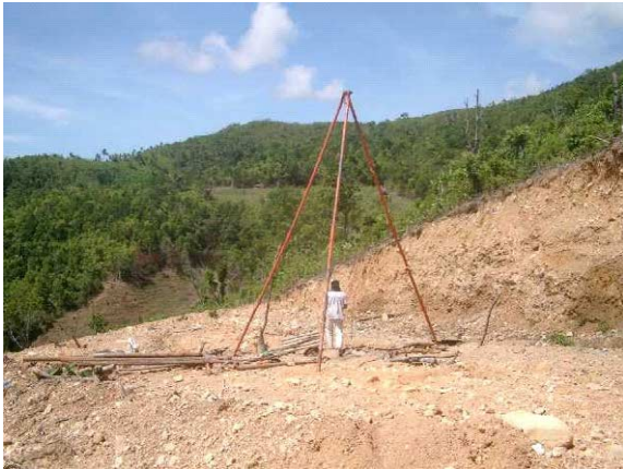
Excavation of Borehole for Geological Investigation
