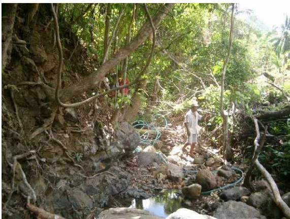
Water Suction for Boring
