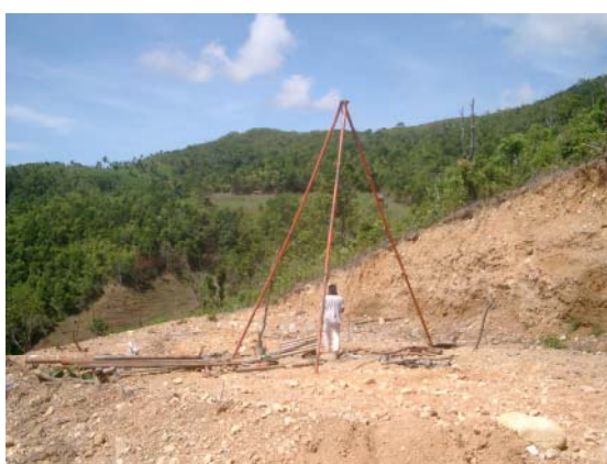
Boring for Geological Survey at the Proposed SLF (June, 2007)
