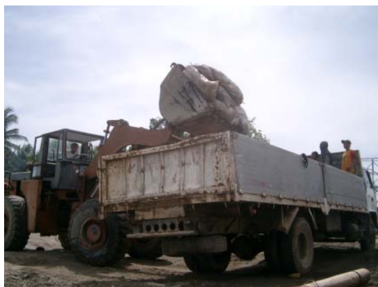
Loading Residual Waste to Dump Truck to Transport to the Proposed SLF (June, 2007)
