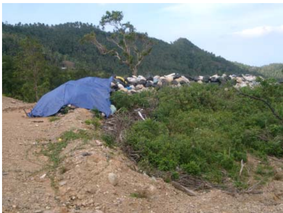
Temporary Stored Residual Waste at the Proposed SLF (June, 2007)
