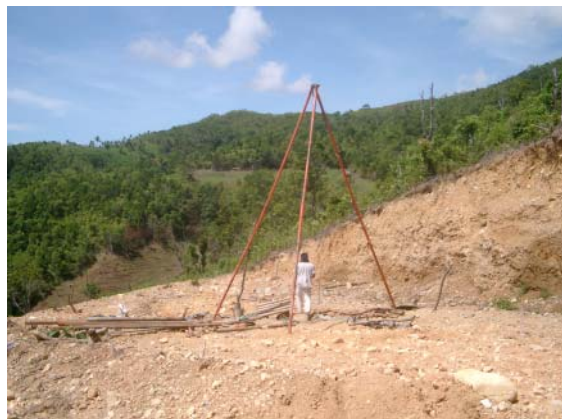
Boring for Geological Survey at the Proposed SLF (June, 2007)
