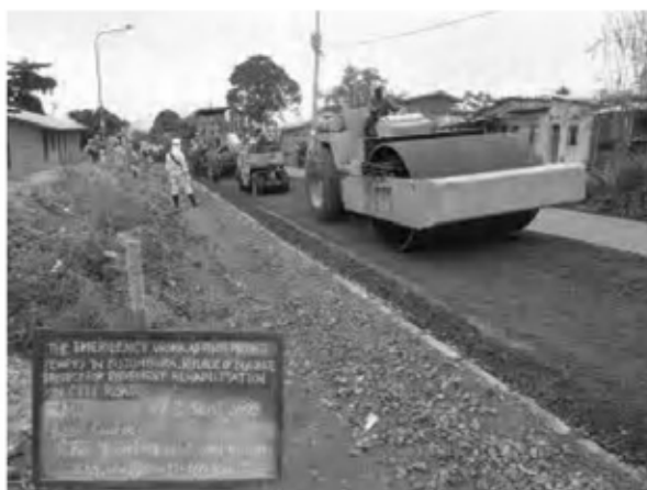
Date : 23/1/2008 ~ 29/1/2008 Activity : Base Course CRS Leveling and Compaction Sta.-0+025 ~ 1+060 Right Side
