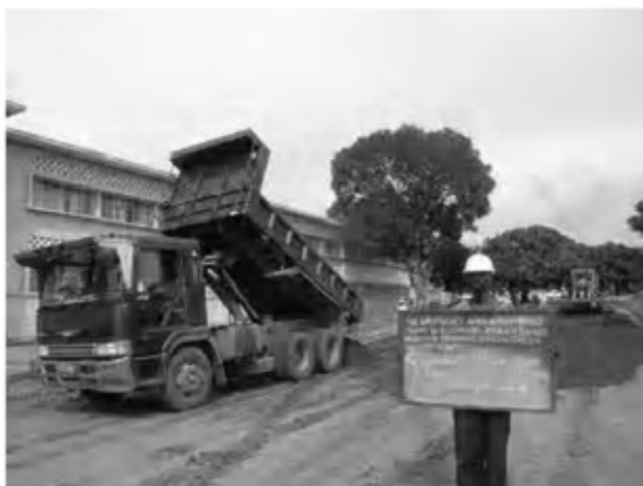
Date : 20/1/2008 Activity : Av. Government Sub-base Murrum Transportation and Dumping
