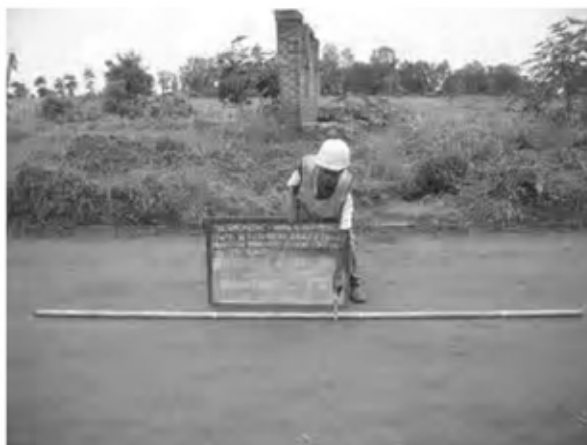
Date : 26 , 29 , 31/1/2008 Activity : RN7 Base Course Quality Control Smoothness Check Sta.-0+025 ~ 1+060 Right Side
