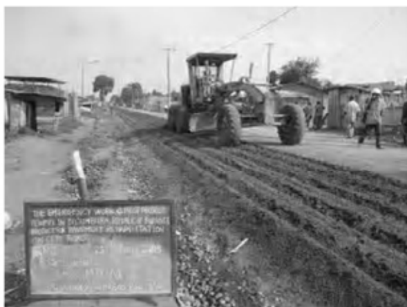
Date : 22/1/2008 ~ 26/1/2008 Activity : RN7 Base Course CRS Mixing Sta.-0+025 ~ 1+060 Right Side
