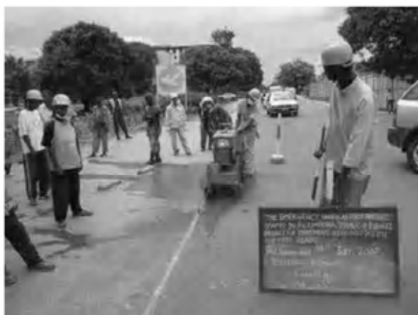
Date : 14/1/2008 Activity : Av. Government Existing Pavement Cutting
