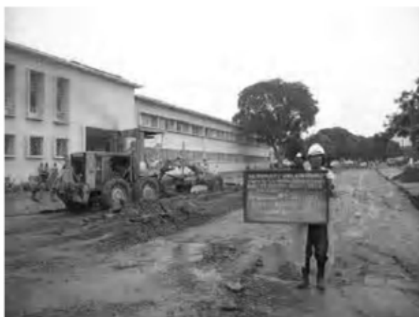
Date : 15/1/2008 Activity : Av. Government Existing Pavement Ripping and Excavation
