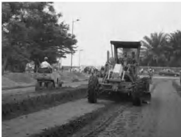
Date : 26/1/2008 Activity : Av. Government Sub-base Mixing and Compaction
