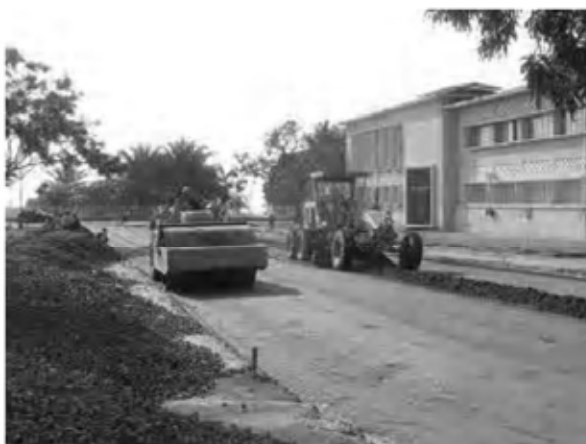
Date : 28/1/2008 Activity : Av. Government Sub-base Leveling and Compaction
