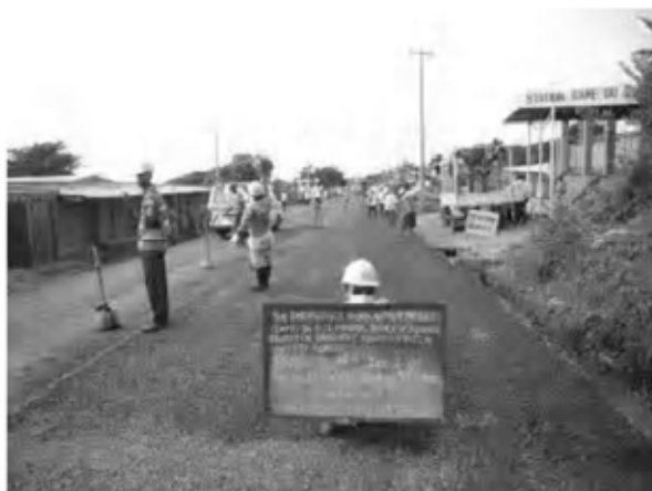
Date : 16/1/2008 Activity : RN7 Double Bituminous Surface Treatment Completion Sta.-0+025~1+660(EP) Left Side
