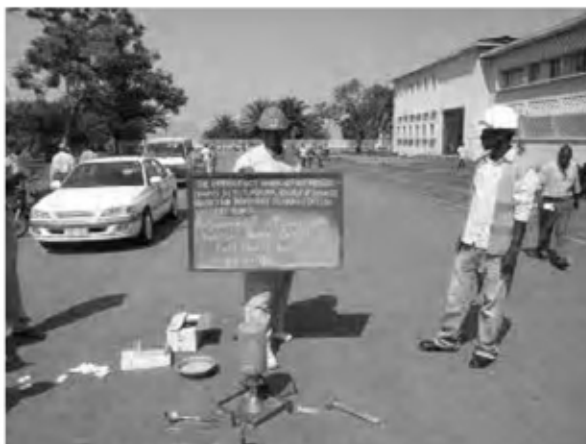
Date : 31/1/2008 Activity : Av. Government Sub-base Quality Control Field Density Test
