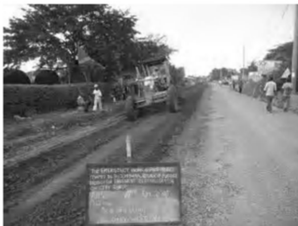
Date : 16/1/2008 ~ 20/1/2008 Activity : RN7 Sub-base Scarification Sta.-0+025 ~ 1+500 Right Side
