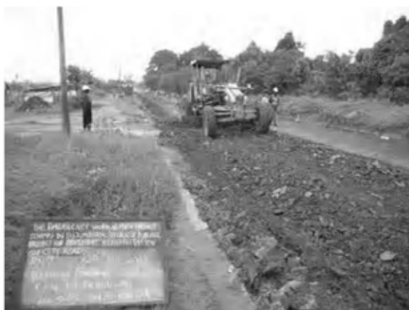
Date : 12/1/2008 ~ 18/1/2008 Activity : RN7 Existing Pavement Ripping and Excavation Sta.-0+025 ~ 1+500 Right Side
