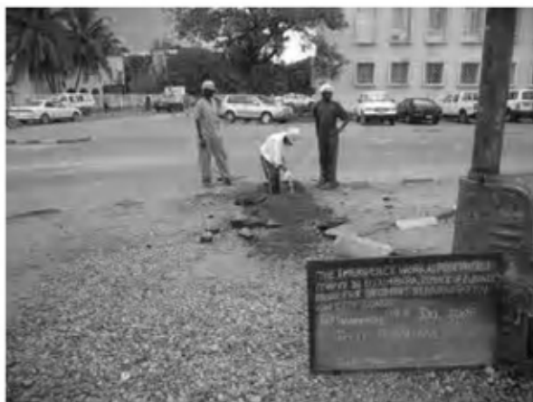
Date : 14/1/2008 Activity : Av. Government Trial Excavation
