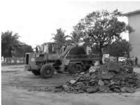
Date : 16/1/2008 Activity : Av. Government Loading the Pavement Dust and Excavation
