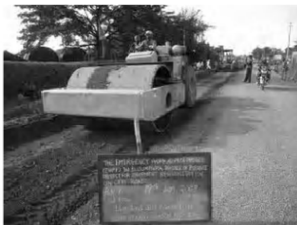
Date : 17/1/2008 ~ 23/1/2008 Activity : RN7 Sub-base Leveling and Compaction Sta.-0+025 ~ 1+500 Right Side
