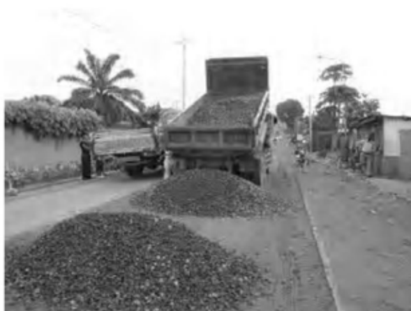
Date : 18/1/2008 ~ 26/1/2008 Activity : RN7 Base Course CRS Dumping and Spreading Sta.-0+025 ~ 1+200 Right Side
