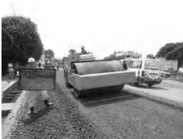
Date : 1/12/2007 ~ 17/12/2007 Activity : RN7 Base Course CRS Rolling Compaction Sta.0+280~1+500 Left Side
