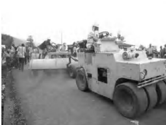
Date : 20 , 21 , 26 , 29/12/2007 Activity : RN7 Double Bituminous Surface Treatment Sweeping the Surface of Base Course Sta. -0+025 ~ 0+240 Left Side Sta. 0+280 ~ 1+500 Left Side
