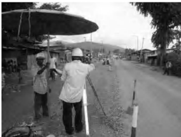
Date : 1/12/2007 ~ 27/12/2007 Activity : RN7 Survey Work for Supporting All Works
