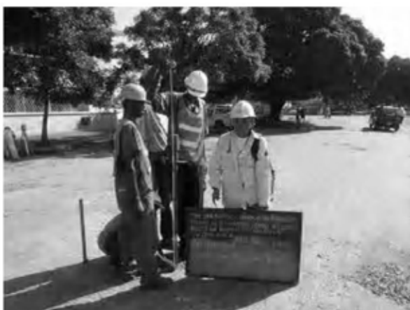
Date : 17/12/2007 Activity : Av. Government Dynamic Cone Penetration Test
