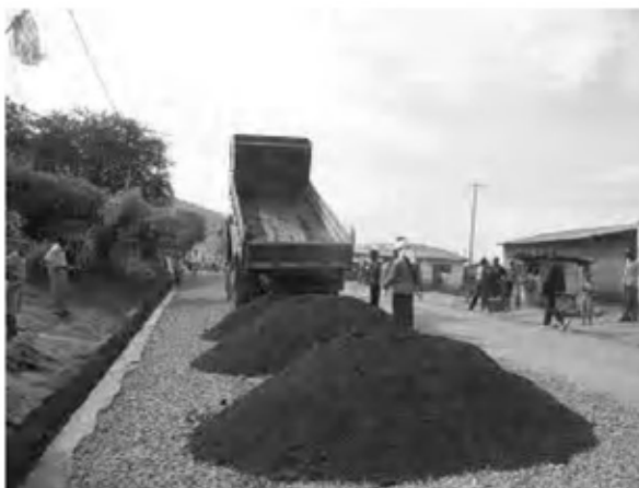
Date : 2/12/2007 ~ 14/12/2007 Activity : RN7 Base Course CRS and Powder Dumping Sta.0+540~1+500 Left Side
