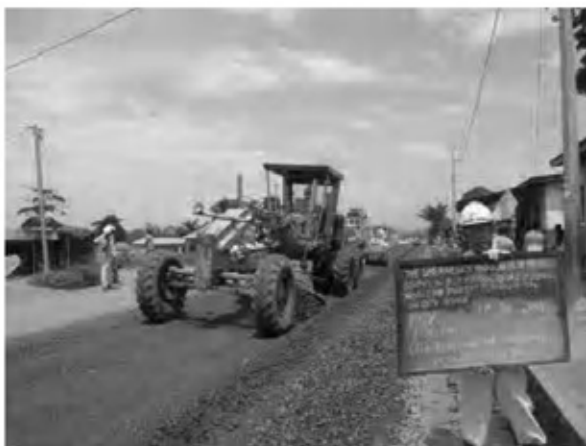
Date : 1/12/2007 ~ 17/12/2007 Activity : RN7 Base Course CRS and Powder Mixing Sta.0+280~1+500 Left Side
