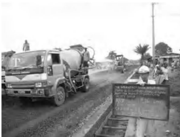
Date : 1/12/2007 ~ 17/12/2007 Activity : RN7 Base Course Moisturizing Sta.0+280~1+500 Left Side
