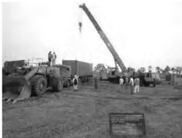
Date : 2/11/2007 Activity : Camp Site Unloading and Setting the Containers
