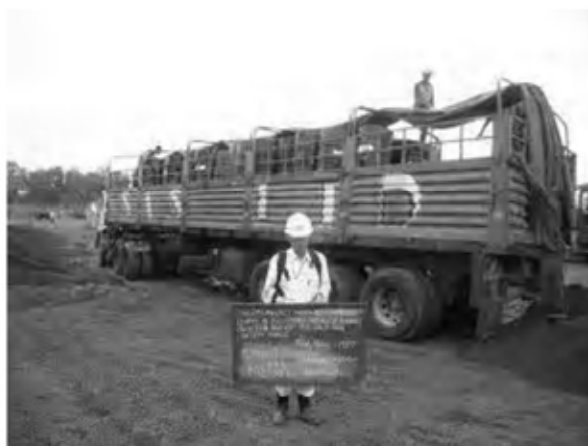
Date : 2/11/2007 Activity : Camp Site Transportation the Materials for Prime Coat MC-30 200ℓ*133drums=26,600ℓ
