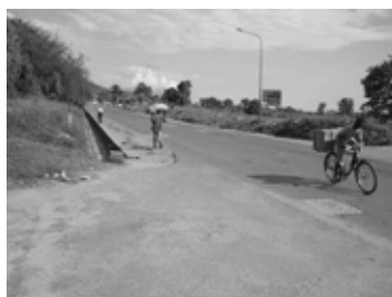
Starting point of the project section (Military Camp Entrance)
