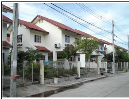
<Constructed houses outside view>
