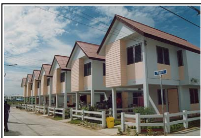
<Constructed houses outside view>
