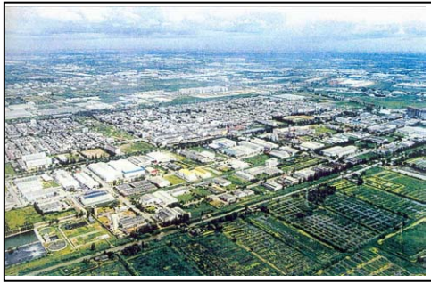
<Bird's eye view of the project site>
