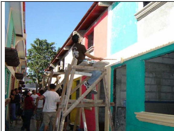
Construction of the Housing
