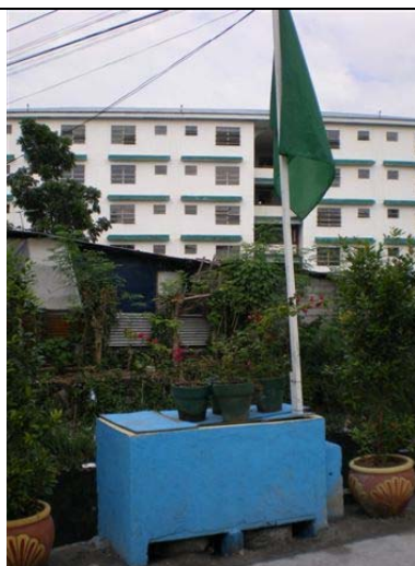
Composting Box under Construction
