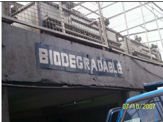
Signage at Waste Storage Area
