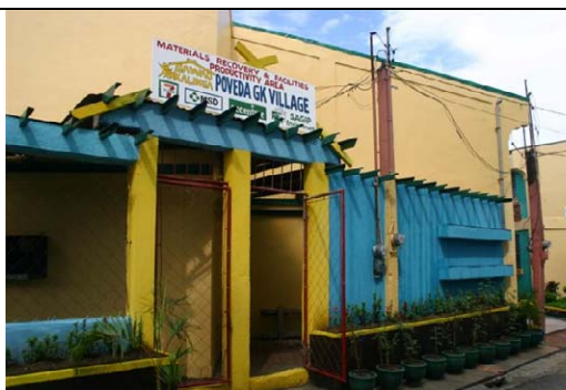
Recyclables Storage Facility
