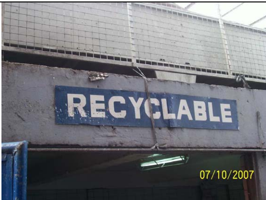
Signage at Waste Storage Area
