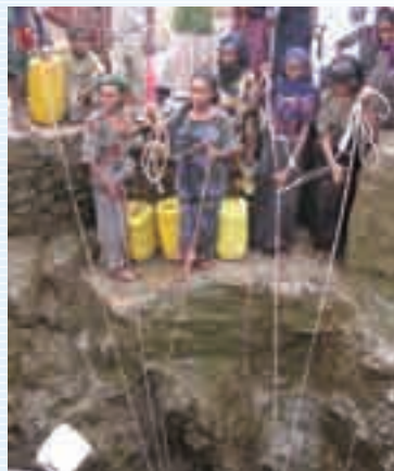
Bailing out water from a hand dug well with a depth of approximately 15 meters
