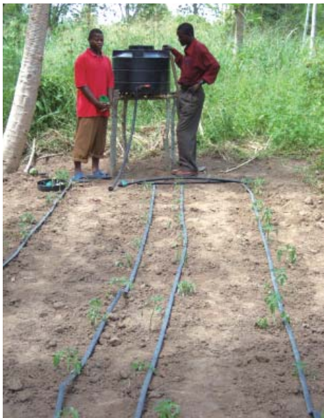
Development of water-saving irrigation technology
